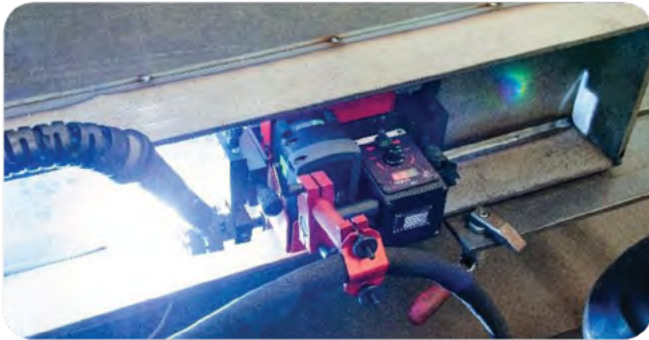
Welding in narrow spaces
