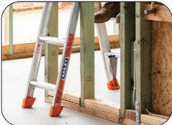
Back legs through studs
