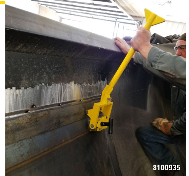
Sheet Alignment with MagPress
